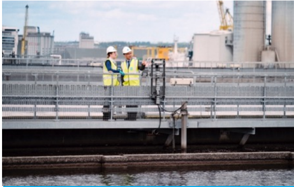
Ringsend Wastewater Treatment Plant
