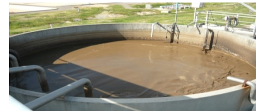
Thickened Sludge Holding Tank
