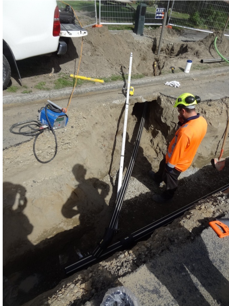
Vacuum Lateral Connection to a Vacuum Main
