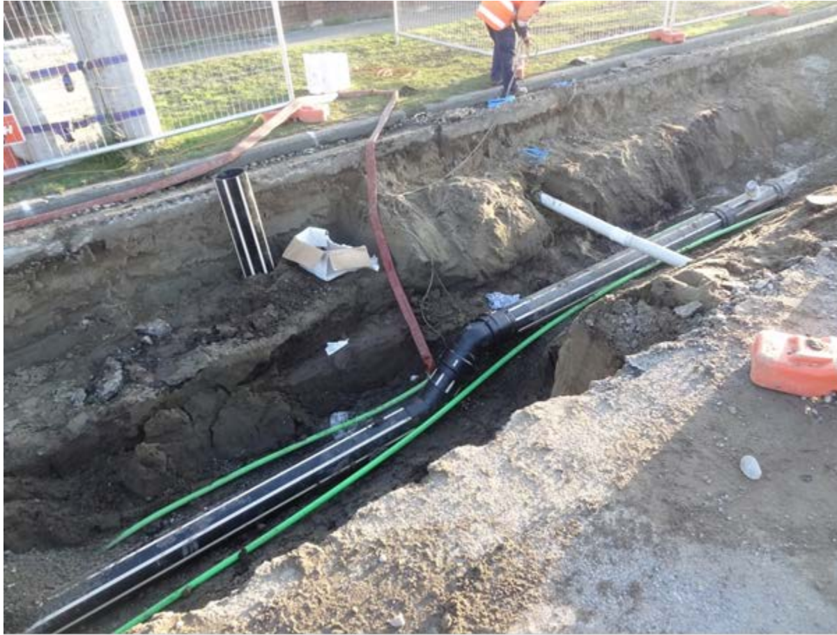
Vacuum Main and Lift Installation
