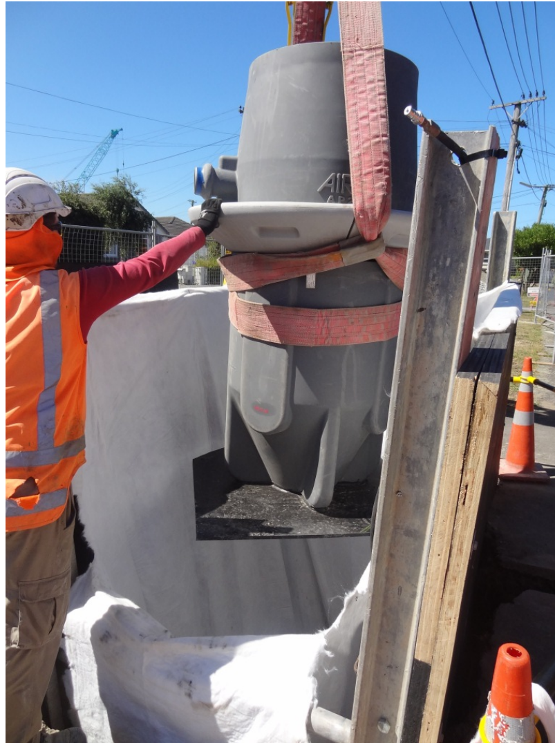
Collection Chamber Installation
