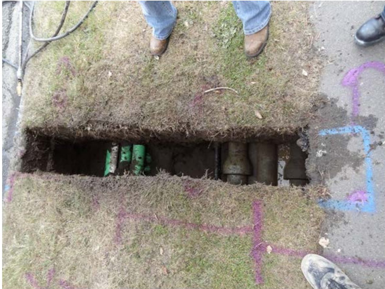
Slot Trench in a Berm
