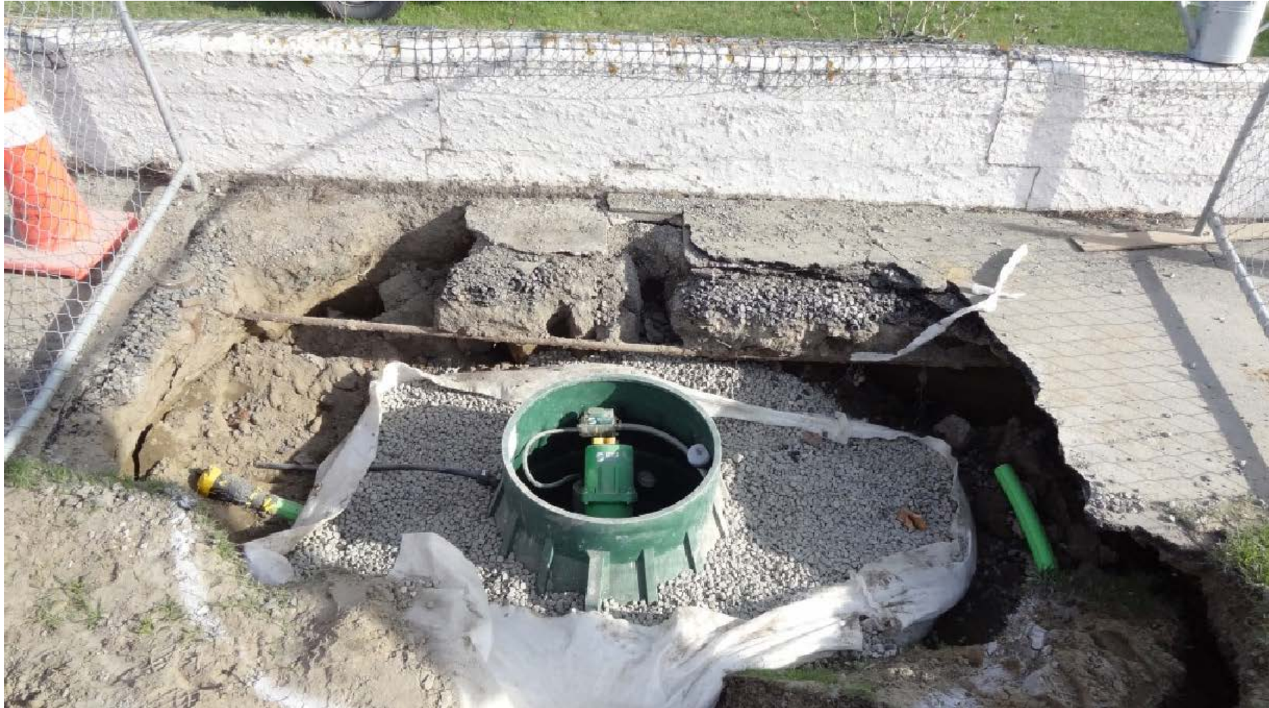
Collection Chamber Installation
