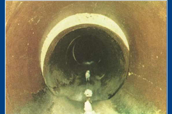
Displaced Joints
