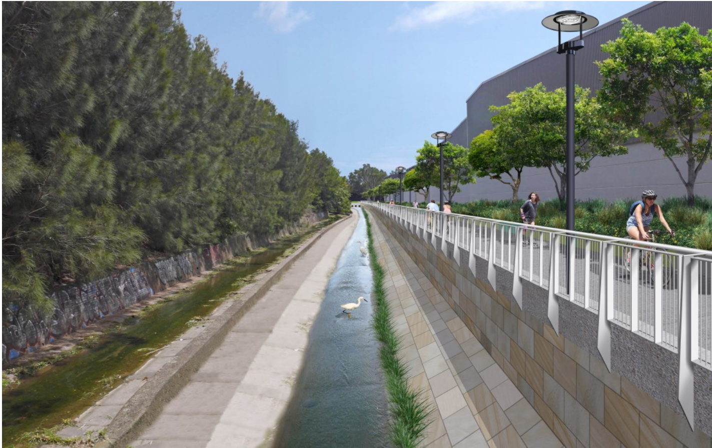
Huntley Street channel widening and shared path
