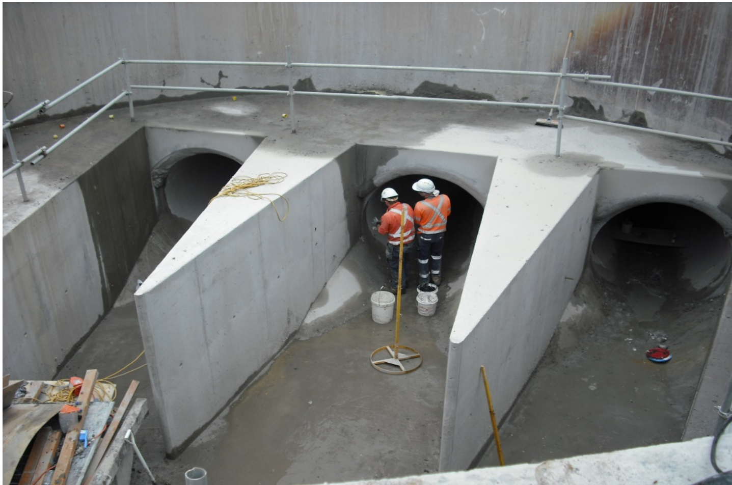
Structure 14 internal benching completion
