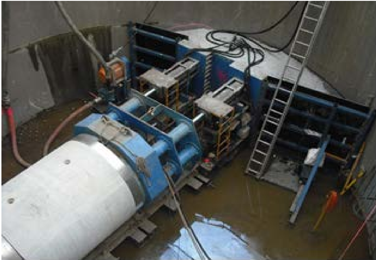
Micro-tunnel installation – DN1800 pipe
