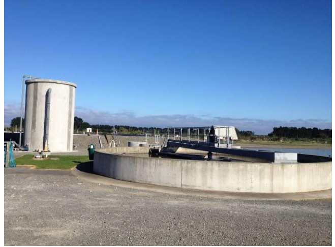
Photograph 1-6: Top Left: Aerated Lagoon; Top Right: Clarifier and Sludge Storage Tank; Middle Left: Secondary Lagoons; Middle Right: Disposal Pipes in Wetland; Bottom Left: Cleared Wetland Area; Bottom Right: Overgrown Wetland Area
