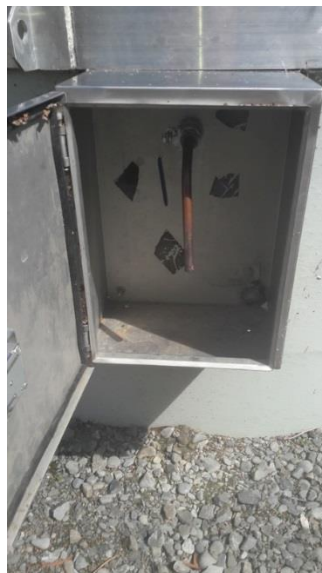
Figure 5: Example of a sample tap outside of the well head
