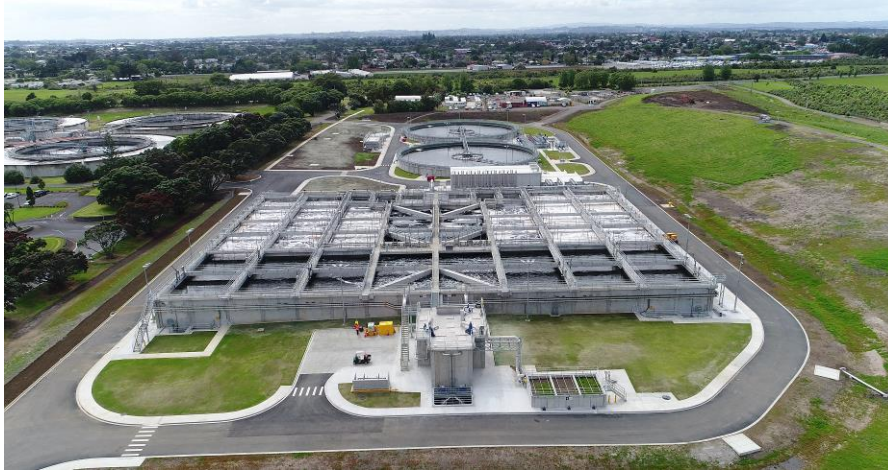
Photograph 1: View of completed MBNRU site from the west
