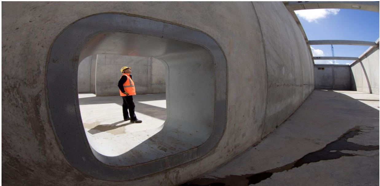
Photograph 8: View through internal access port/door in reactor
