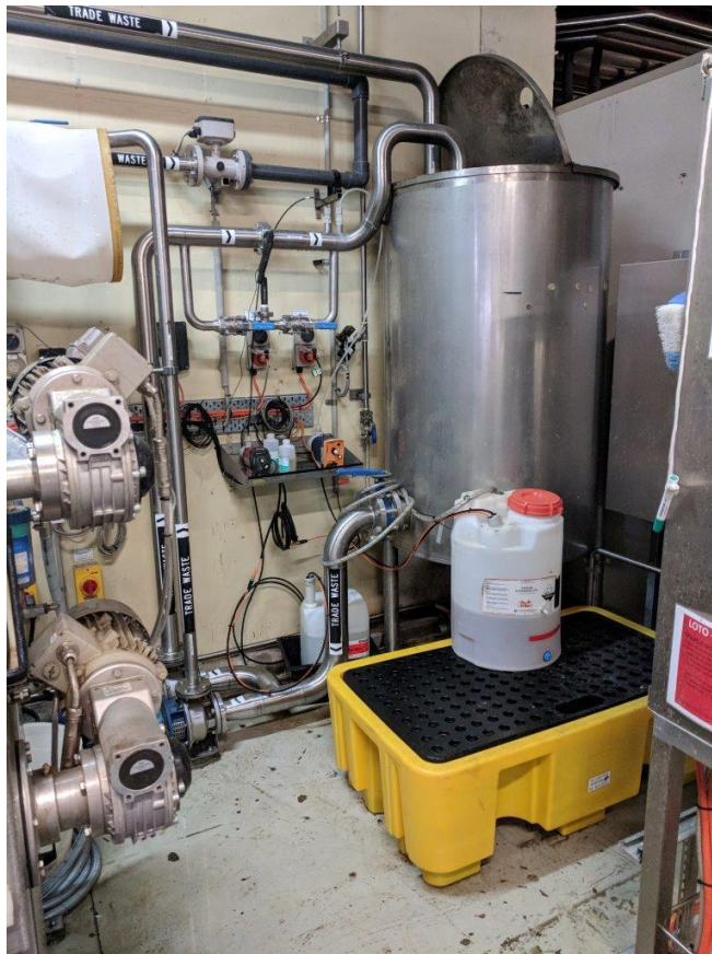
Photograph 2: Inlet buffer tanks (background) and Salsnes™ filter (foreground)
