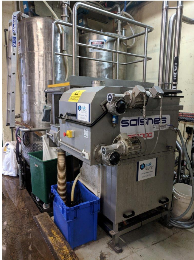
Photograph 2: Inlet buffer tanks (background) and Salsnes™ filter (foreground)
