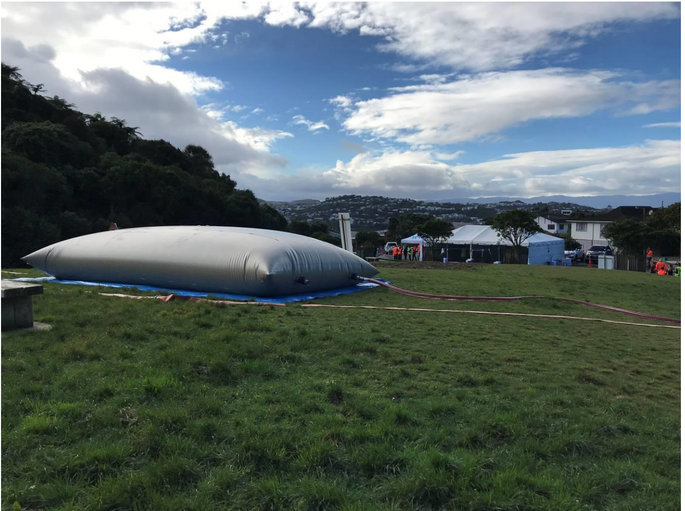
Figure 8 – Filled 20,000L Treated Water Storage Bladder
