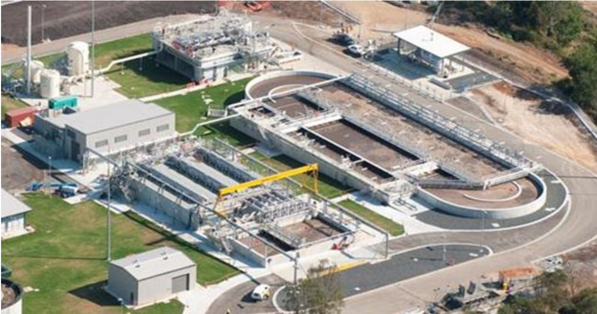
Figure 2. Goodna STP MBR, 90,000EP, Brisbane Australia.
