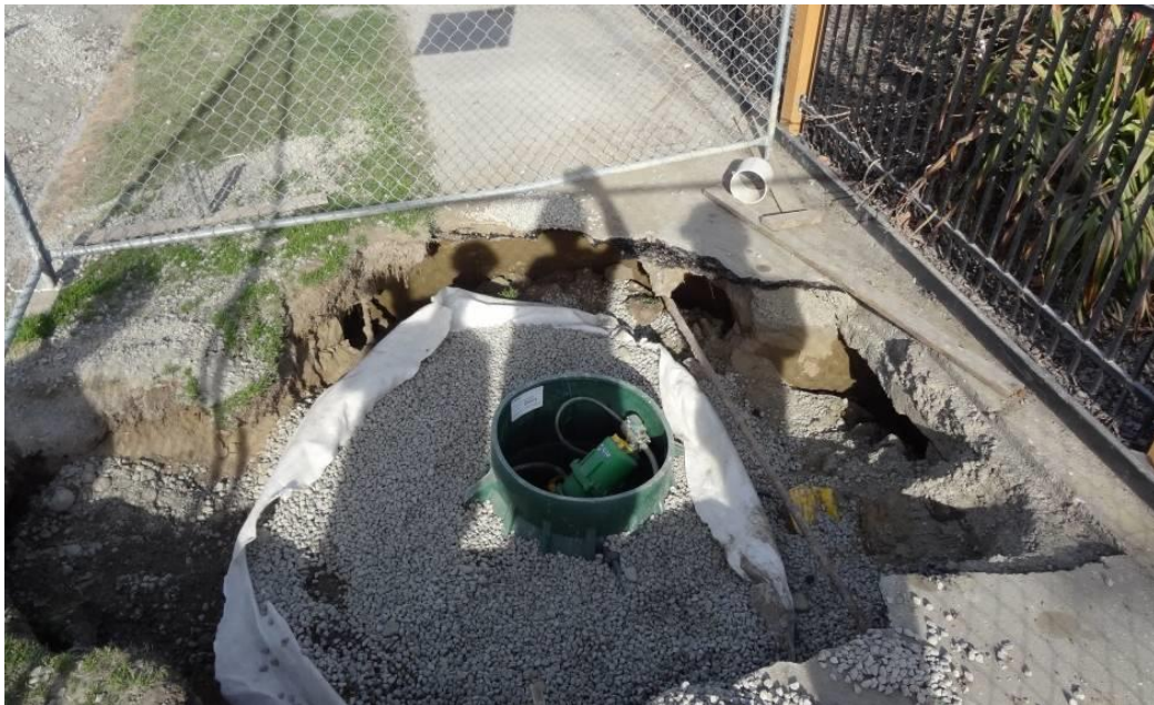
Figure 3 Vacuum Main and Lift Installation
