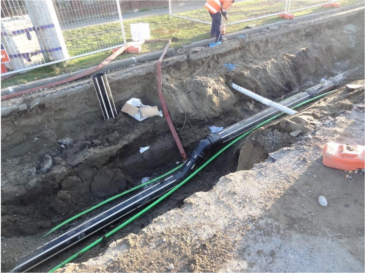
Figure 3 Vacuum Main and Lift Installation
