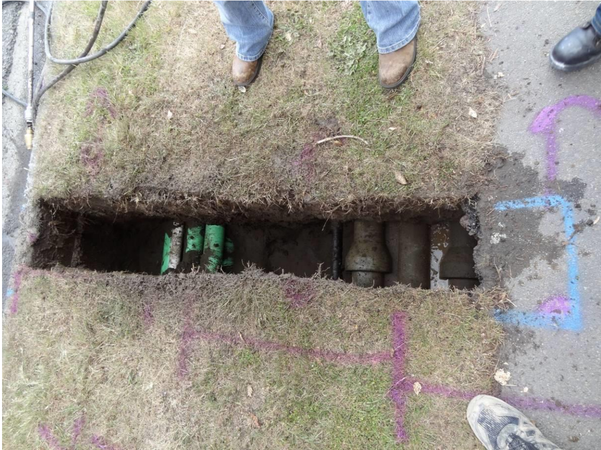
Figure 9 Existing Services in the Berm Potholed Prior to Location of a Collection Chamber
