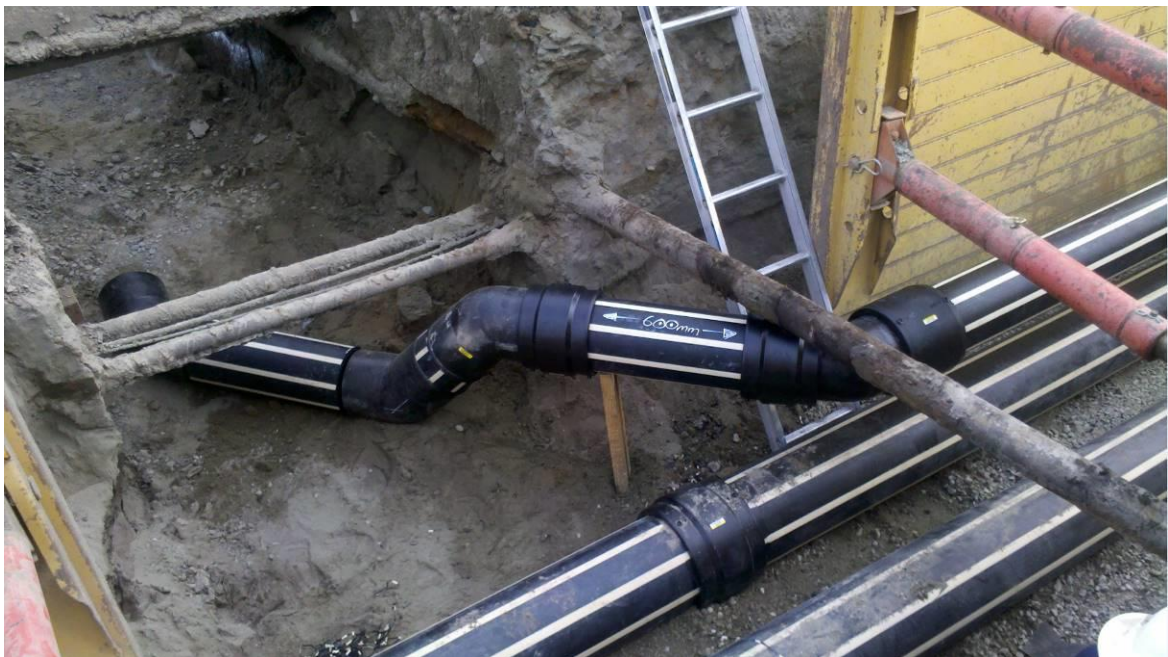
Figure 9 Existing Services in the Berm Potholed Prior to Location of a Collection Chamber
