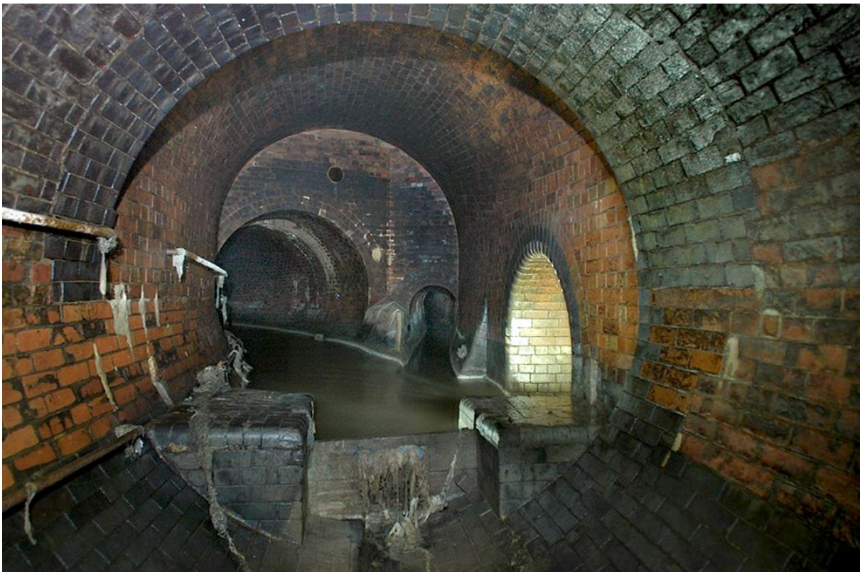
Photograph 1: Bazalgette’s 19 th Century Ranelagh Sewer
