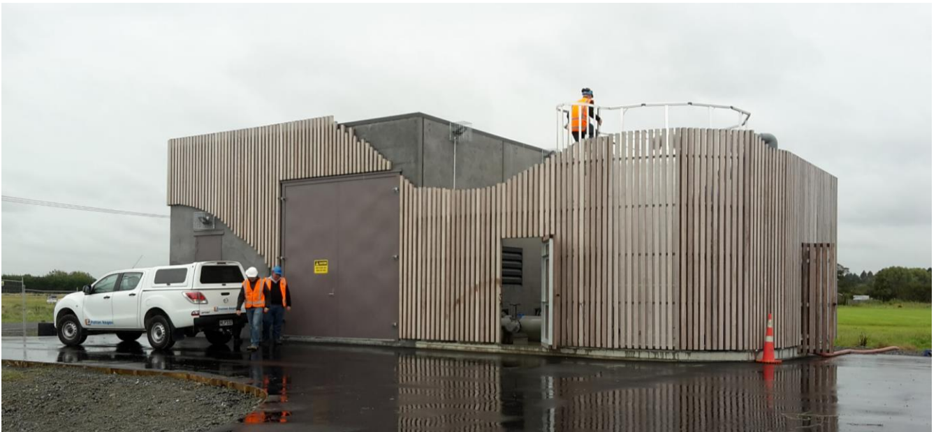
Figure 3: PS104 nearing completion
