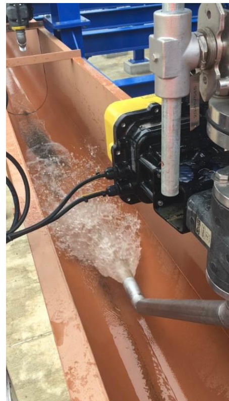
Photograph 10: Purge operation with 45° bends installed on the purge valve outlets
