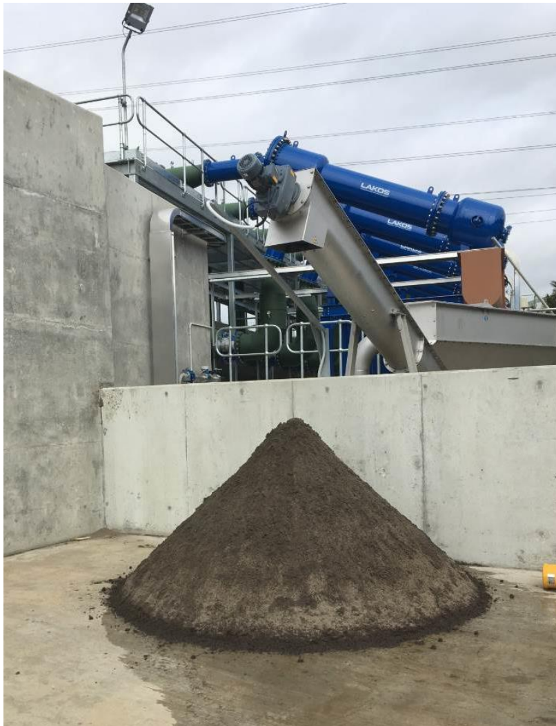
Photograph 12: Sand collection bay
