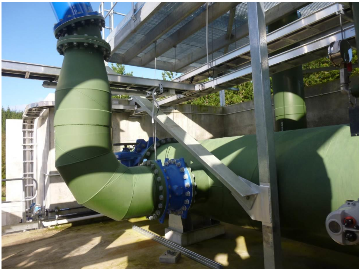
Photograph 11: Diagonal cross bracing installed on the sand separation system platform structure
