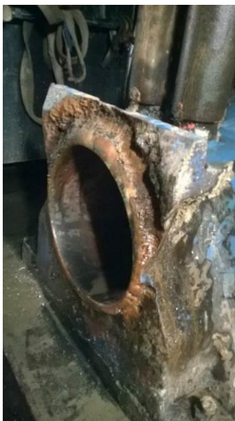
Photograph 3: Abraded pedestal face from sand wear
