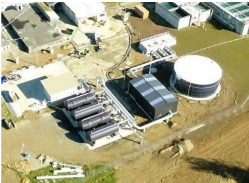
Photograph 2: Branxholme WTP aerial photograph showing the major plant extent inclusive of the GAC filters
