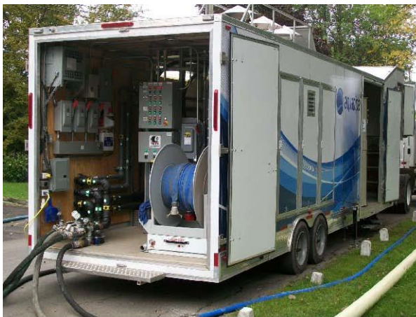
Figure 18: Curing with hot water
