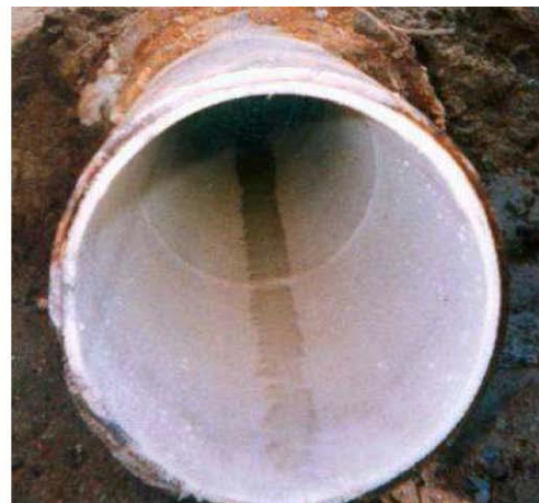
Figure 19: Pipe rehabilitated with AQUA-PIPE®
