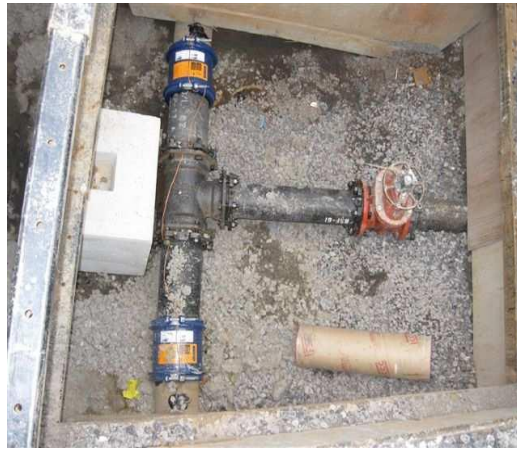
Figure 22: Typical reconnection in an insertion pit
