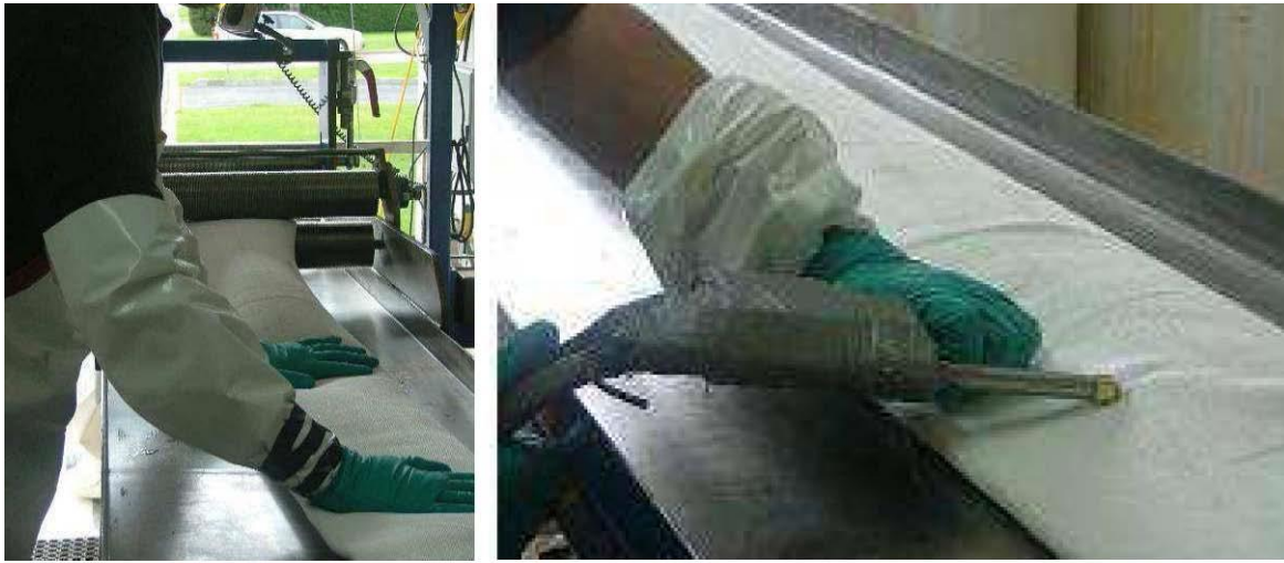
Figure 14: Impregnation of the liner
