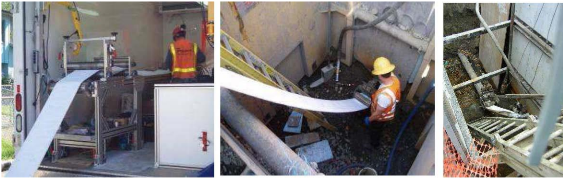
Figure 16: Insertion of the liner
