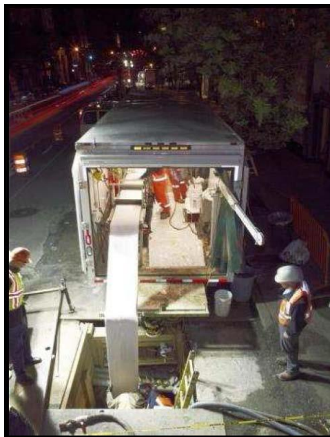
Figure 15: Insertion of the liner
