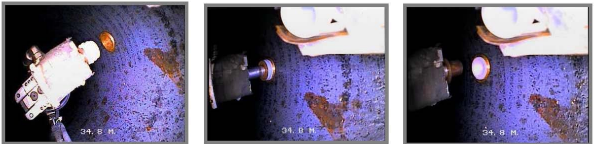
Figure 12: Plugging service connections
