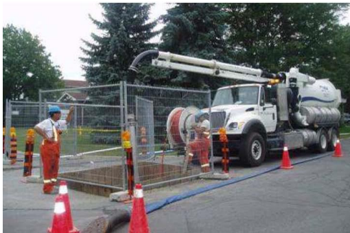
Figure 6: Trench box and fencing
