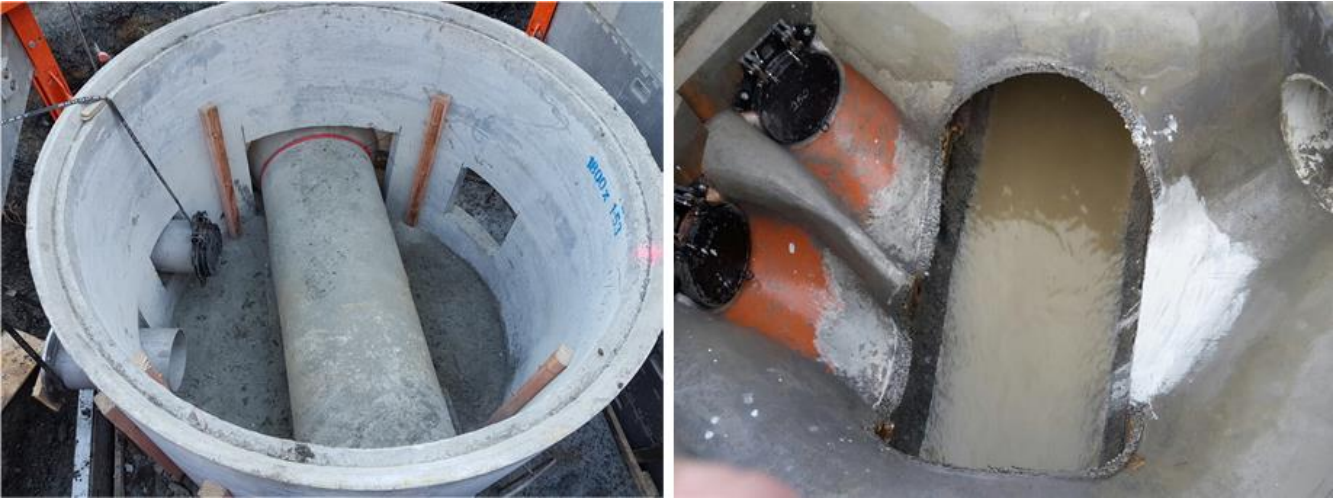
Figure 12: Building a manhole over live sewer assets.
