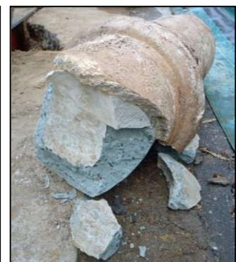
Picture 11: Pipe filled with concrete
