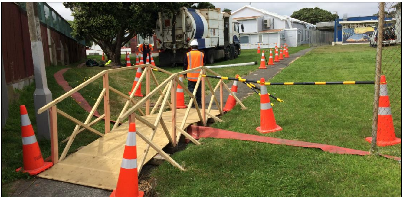
Figure 10: Bridged walkway constructed to manage over pumping alignment.
