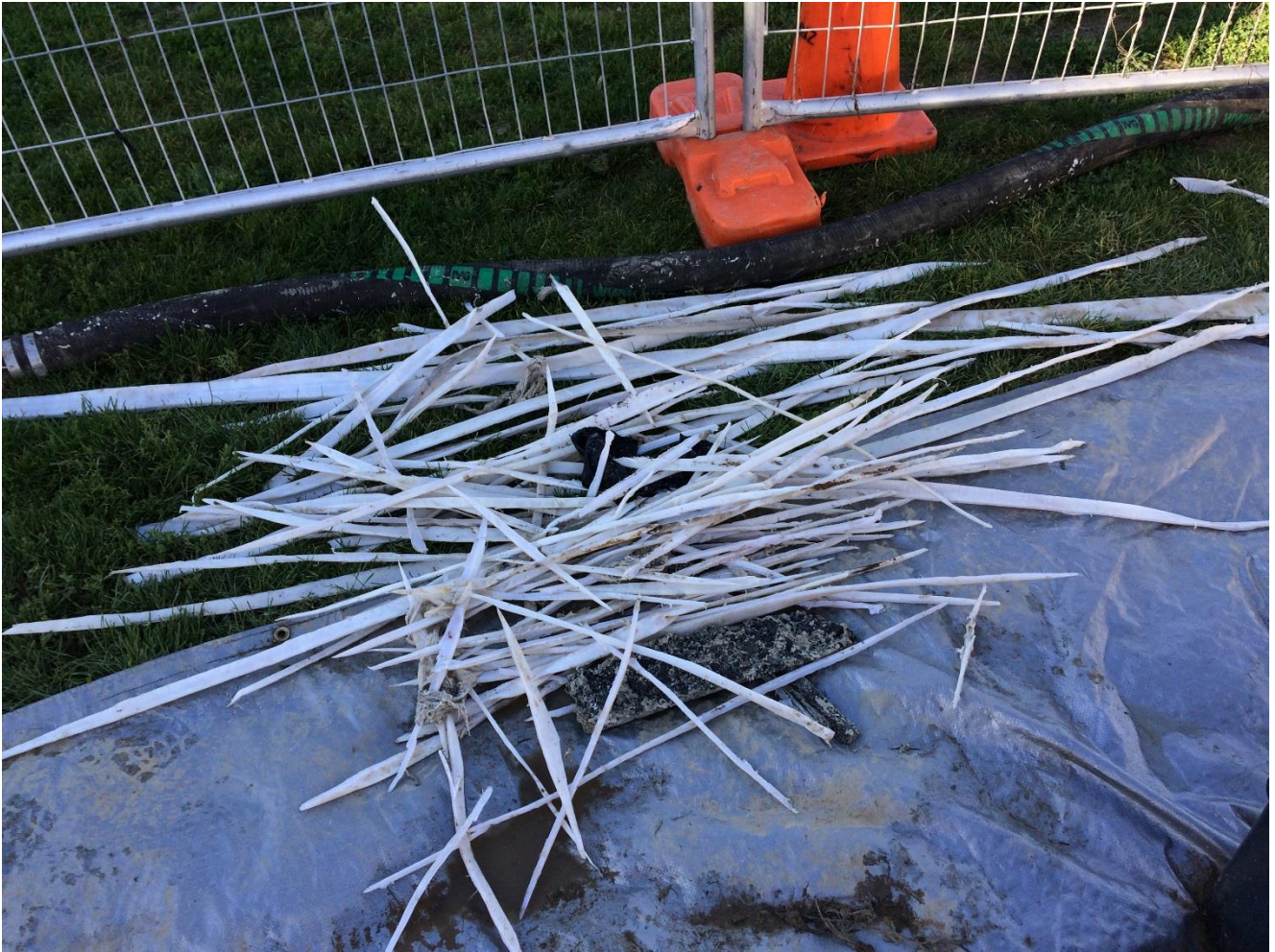
Figure 13: Cut liners removed from the U-Shaped Pipeline.
