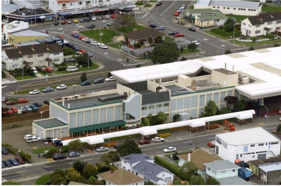
Figure 4 – Waterloo Water Treatment Plant
