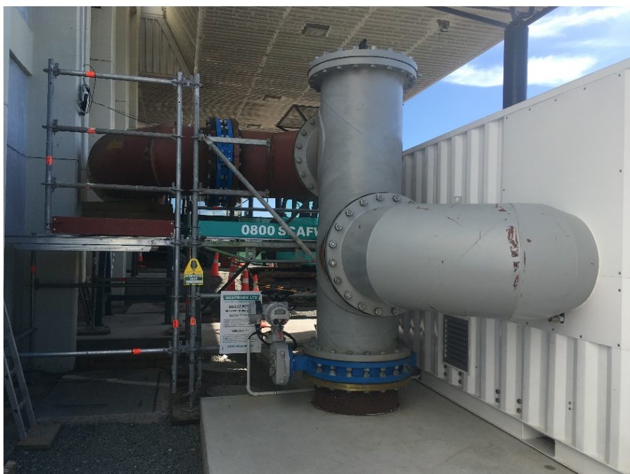
Figure 11 – Installation of UV1 at Waterloo WTP
