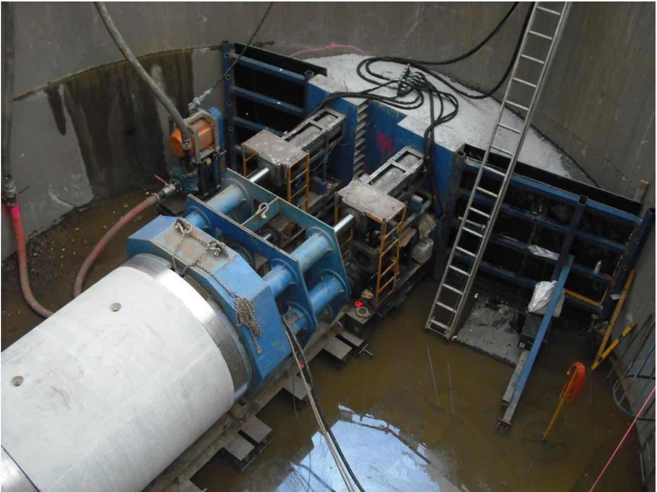
Photograph 3: Microtunnel installation DN1800 pipe
