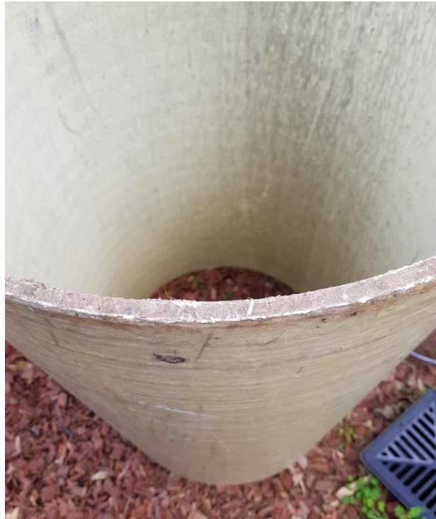
Figure 4 A side picture of the GRP pipe imaged
