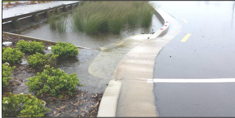
Figure 14 : Rain Garden Kerb Entry
