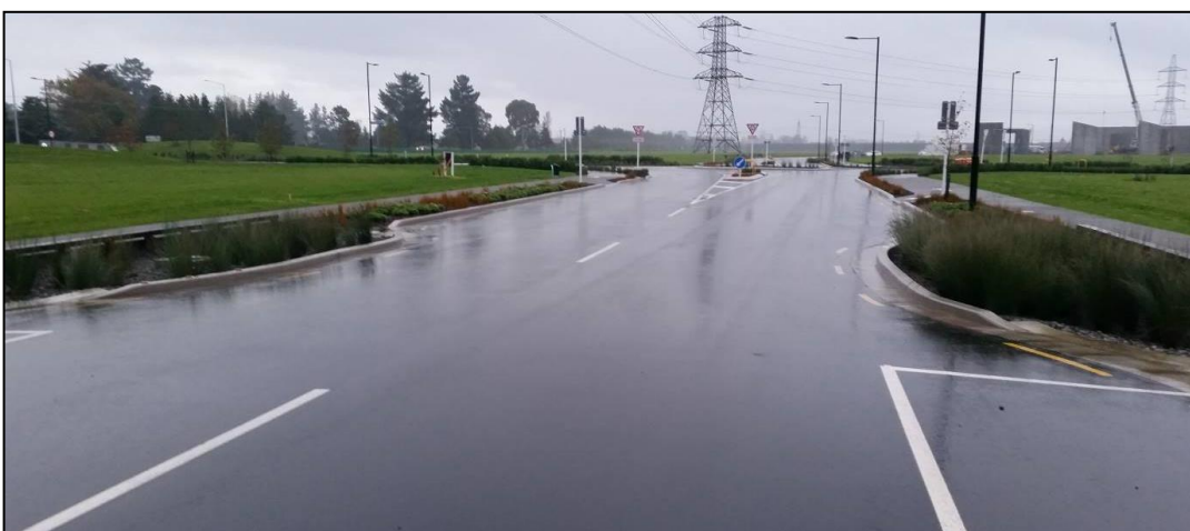
Figure 5: Photo of rain gardens in streetscape
