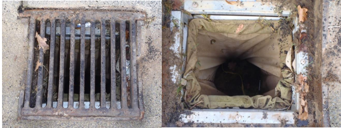
Plates 3-6. Above, a catchpit grate on the concrete path (left, Plate 3) and the Enviropod filter bag (right, Plate 4). Below, crumb rubber deposited within the Enviropod filter bag overflow (left, Plate 5) and in the bottom of the bag (right, Plate 6)
