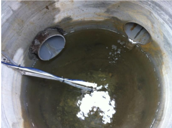
Plate 1 (left): View inside the manhole where monitoring equipment was located. Exit pipe orifice is top left, one sub-surface drain can be seen entering at top right.
