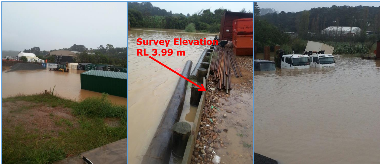
Photographs 3, 4 & 5: Flooding during March 2017 (Courtesy of Ron Stevenson).
