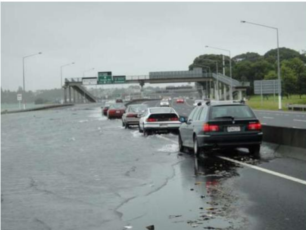
Fig 3 SH1 Esmonde Road to Northcote, Auckland, Jan 2011 (source: Peter Mitchell, Auckland Motorway Alliance)
