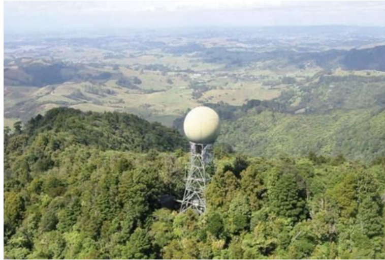
Figure 1: The MetService radar near Warkworth.
