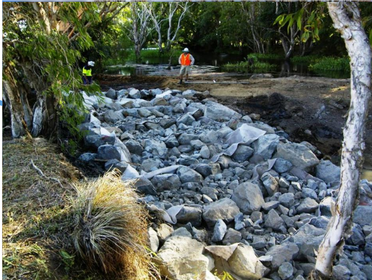
Rock-ramp weir design
