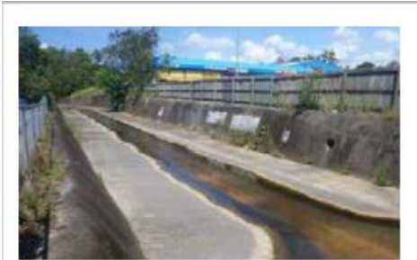
Existing Condition : Concrete Channel
