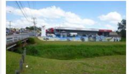
Existing Condition : Grassed Channel
