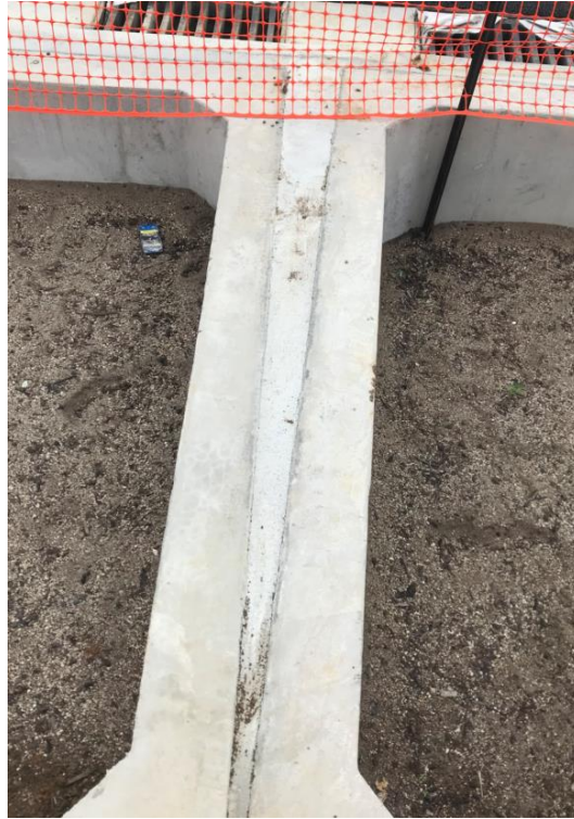
Figure 17: Concrete fill between raingarden surrounds
