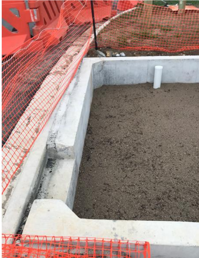
Figure 15: As-built pre-cast raingarden surround
