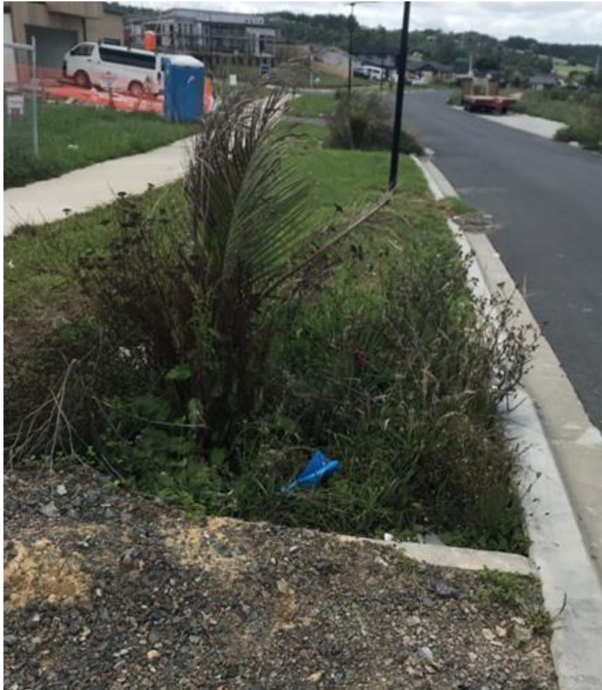
Figure 21: Unmaintained Raingarden
