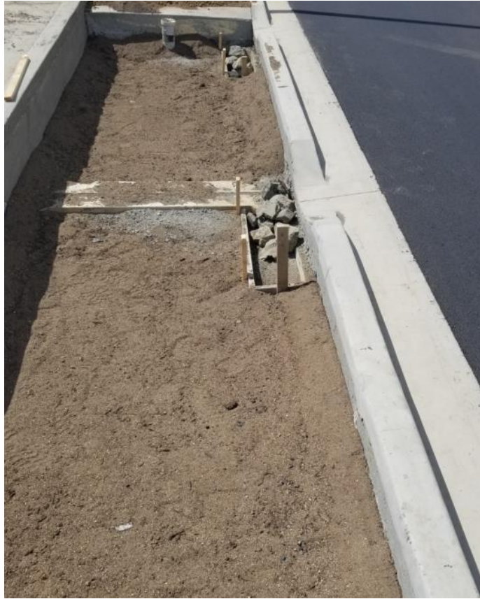
Figure 16: Kerb and Channel above raingarden surround
