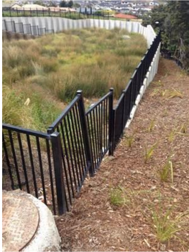
Figure 7: Central Bioretention Raingarden
