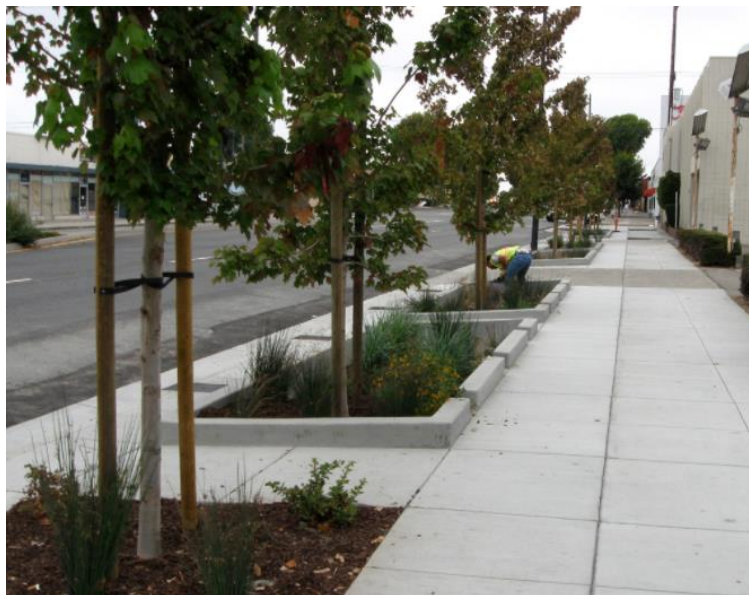
Figure 6: At source Bioretention Raingarden
