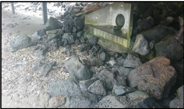
Photograph 1 and 2: Combined Sewer Overflow and debris resulting from its operation in St Marys Bay at low tide
