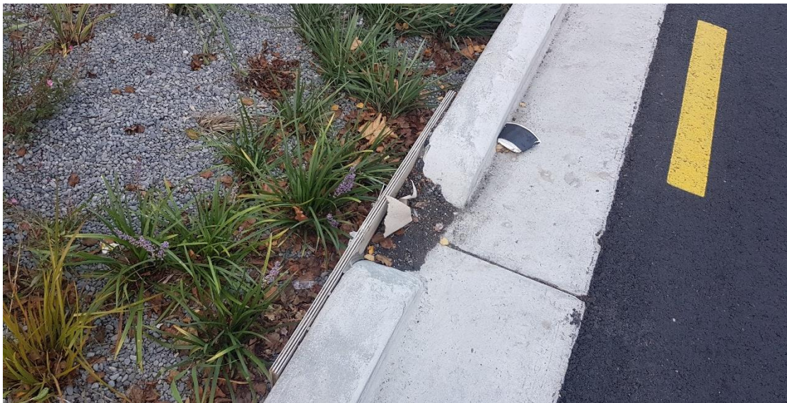
Figure 14: Temporary barrier to prevent construction sediment entering new rain garden
