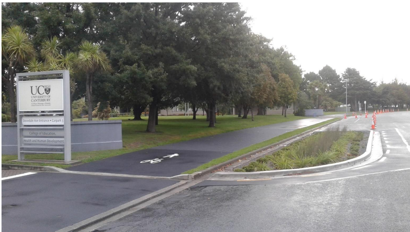
Figure 5: Rain garden installed as part of cycle route development, Christchurch
