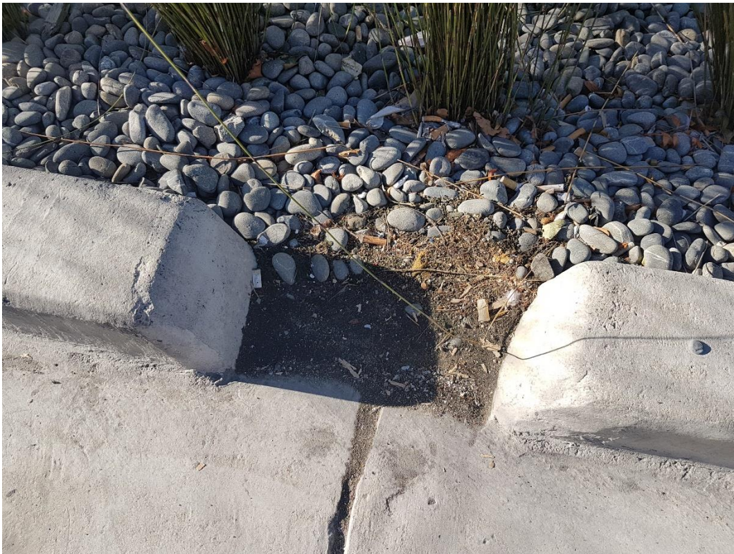
Figure 10: Mulch placed at or above the inlet level
