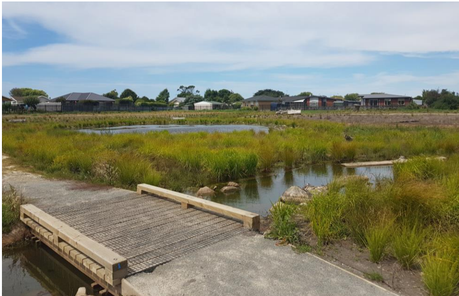
Photograph 3: The Constructed Te Oranga Waikura Urban Forest (photo: WSP-Opus)
