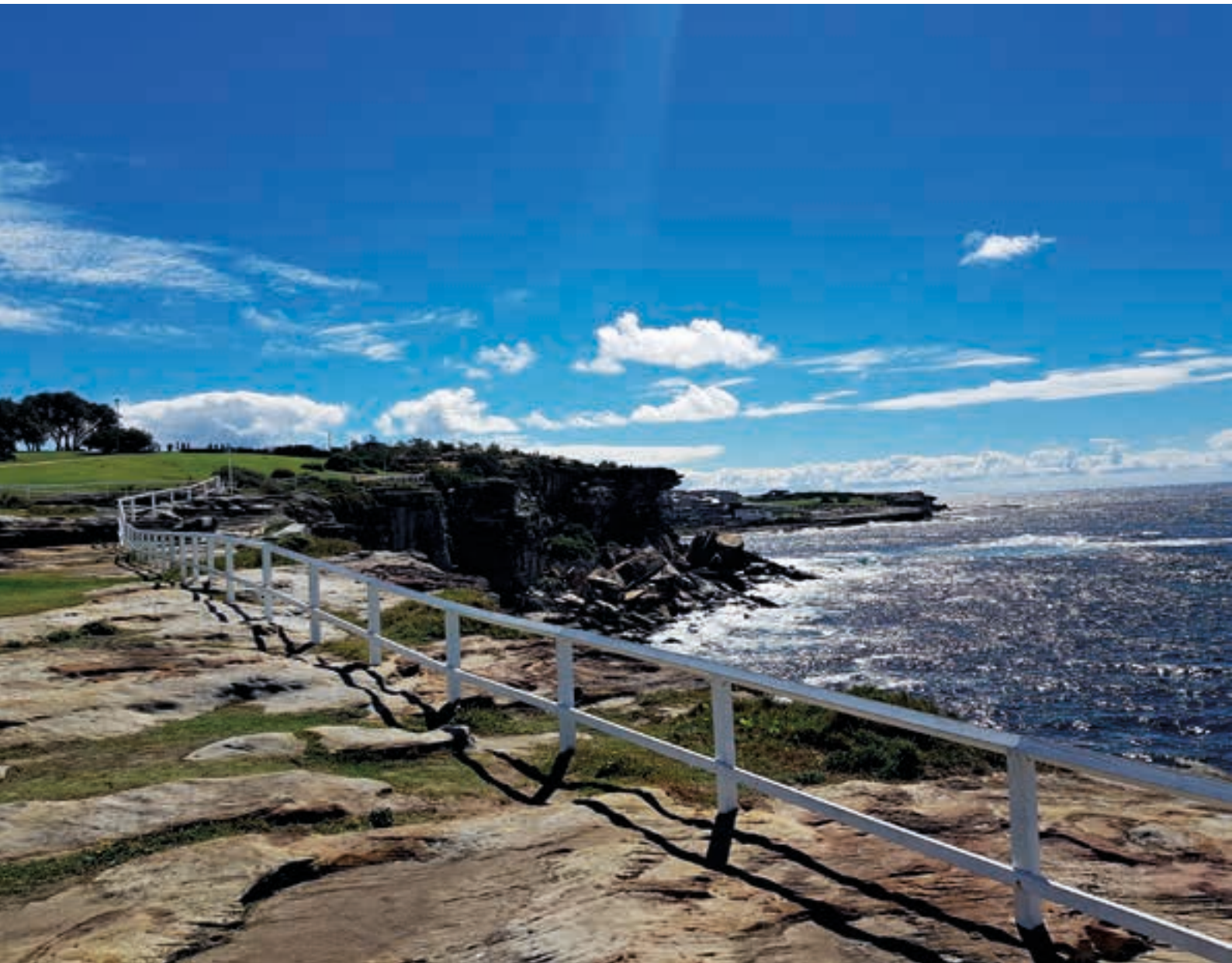
Even without the predicted modeling of sea level increases, coastal erosion is a natural but harsh reality for a country built on soft sedimentary rock. Even on the Australian east coast this receding sandstone cliff at Coogee Beach in Sydney is forever crumbling into the sea due to the action of the sea.
