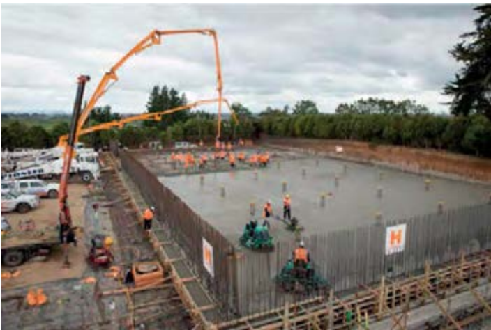
First pour of 950m 3 showing two concrete pump cranes.
