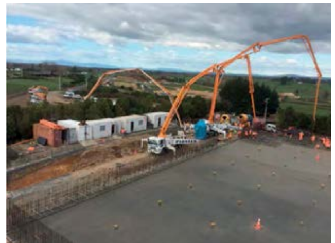
Second pour of 950m 3 showing the over pump configuration.
