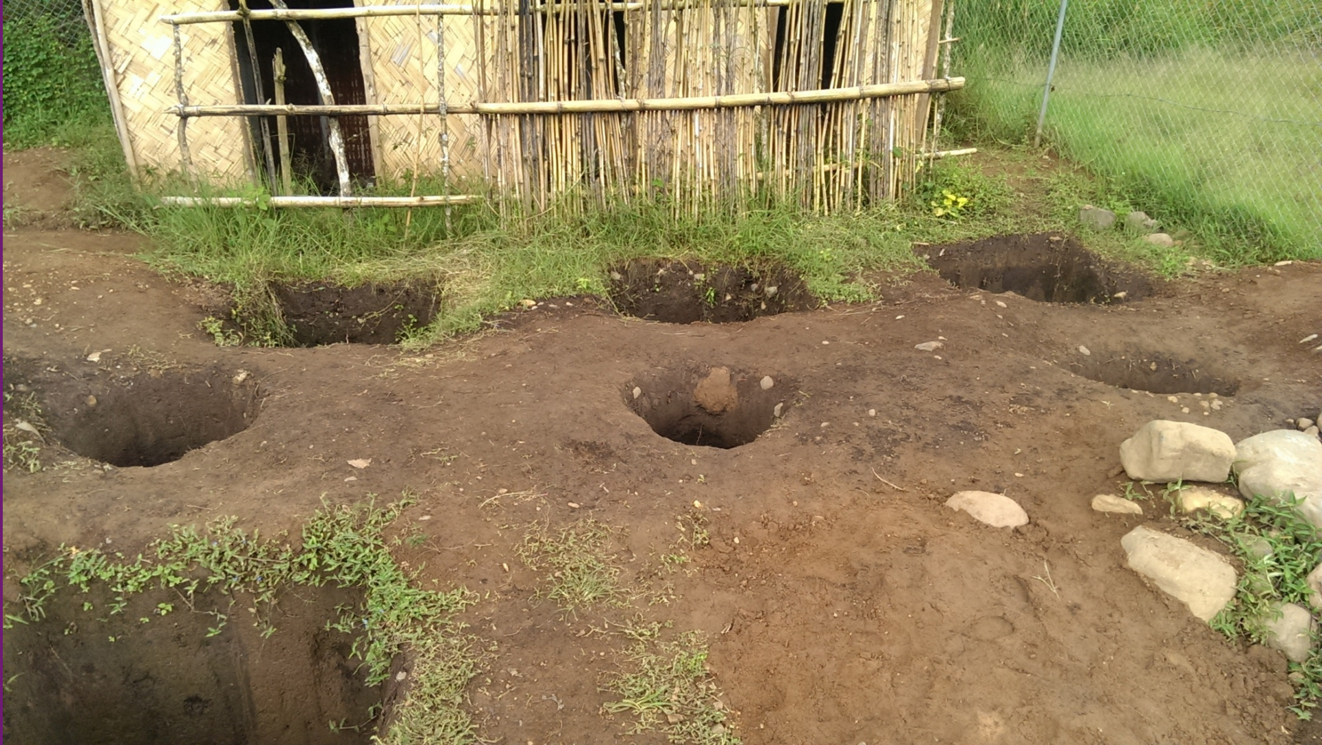
Freshly dug pits where toilets will be built
