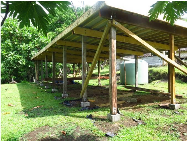
Photograph 1 & 2: Examples of the Wawan project rainfall harvesting structures near the end of construction.
