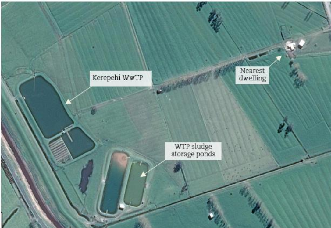
Figure 3: Kerepehi Wastewater Plant and Tanners Ponds
