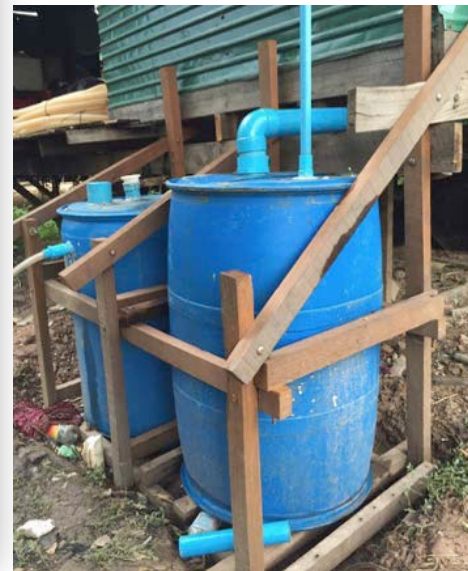
Household sized HandyPod systems on seasonally floating household adapted for dry and wet season
