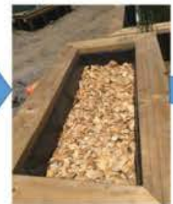
Woodchip Denitrification Filter for residual nitrate removal via disinfection
