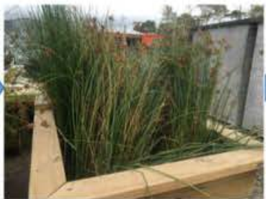
Surface Flow Constructed Wetland (SFCW) for further organic compounds and nutrient removal
