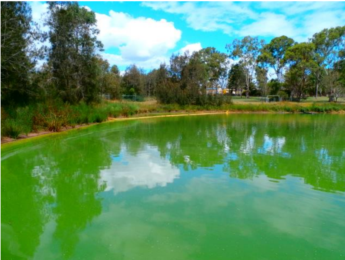
Photograph 1 – A Wastewater Effluent Storage Lagoon in SE Queensland, prior to dosing of the product, Diatomix.
