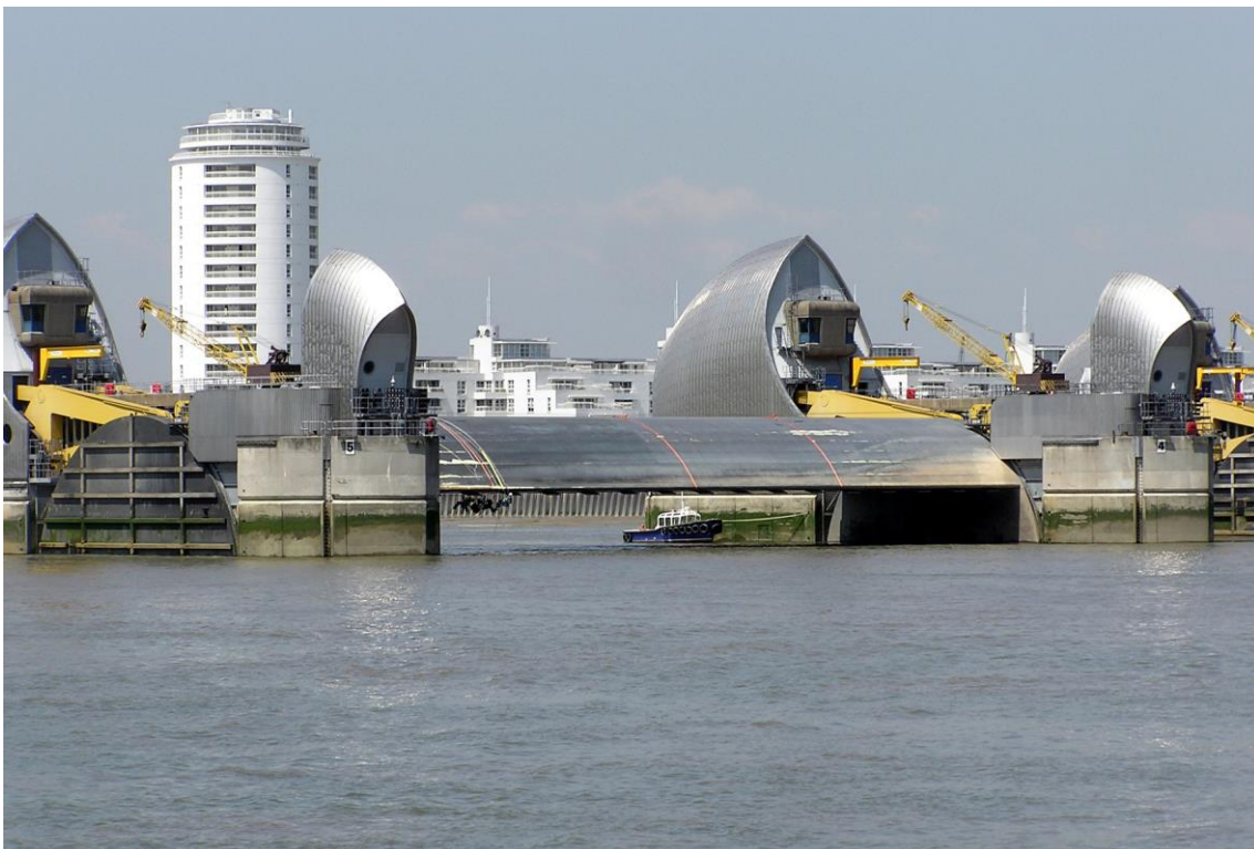
Figure 2 The Thames Barrier
