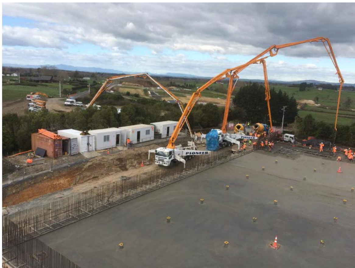
Photo 2: Second pour of 950m 3 showing the over pump configuration
