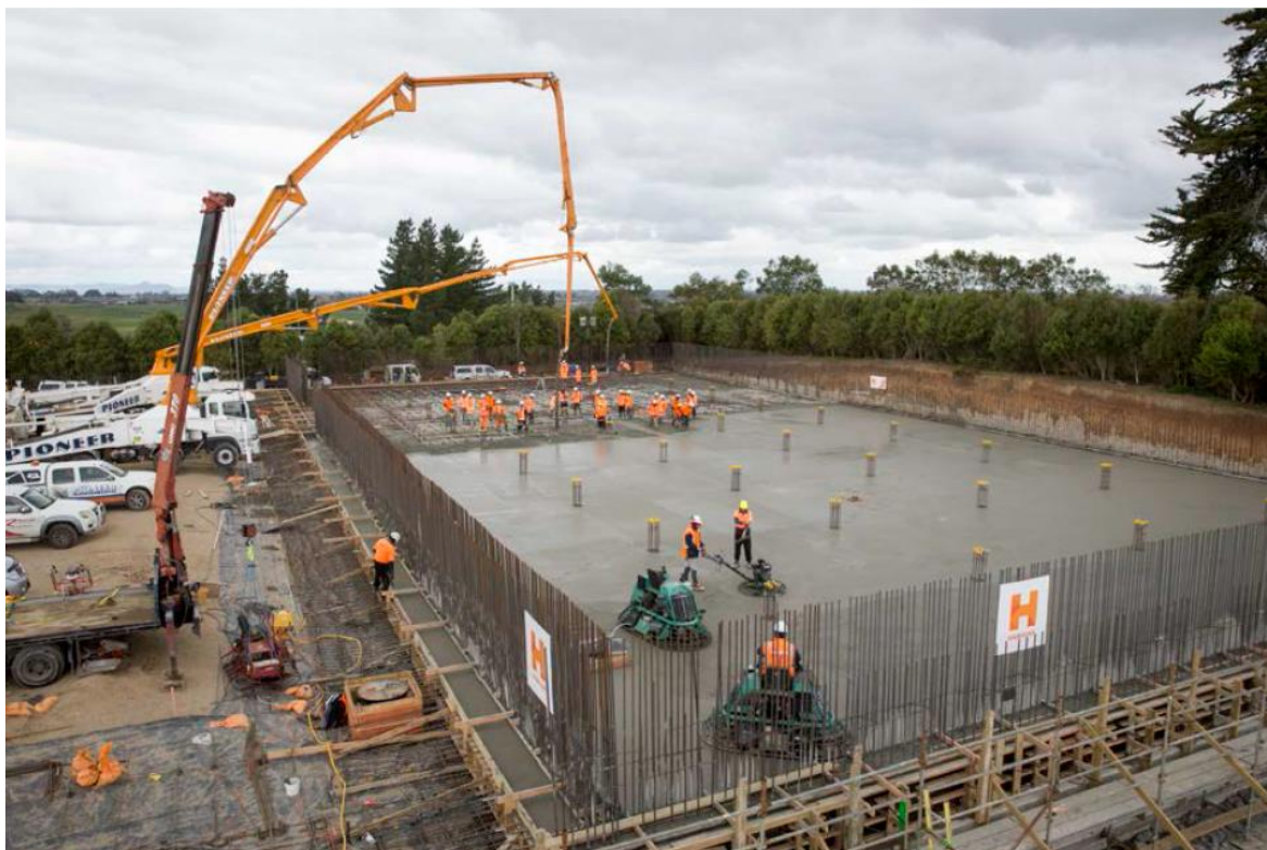
Photo 2: Second pour of 950m 3 showing the over pump configuration
