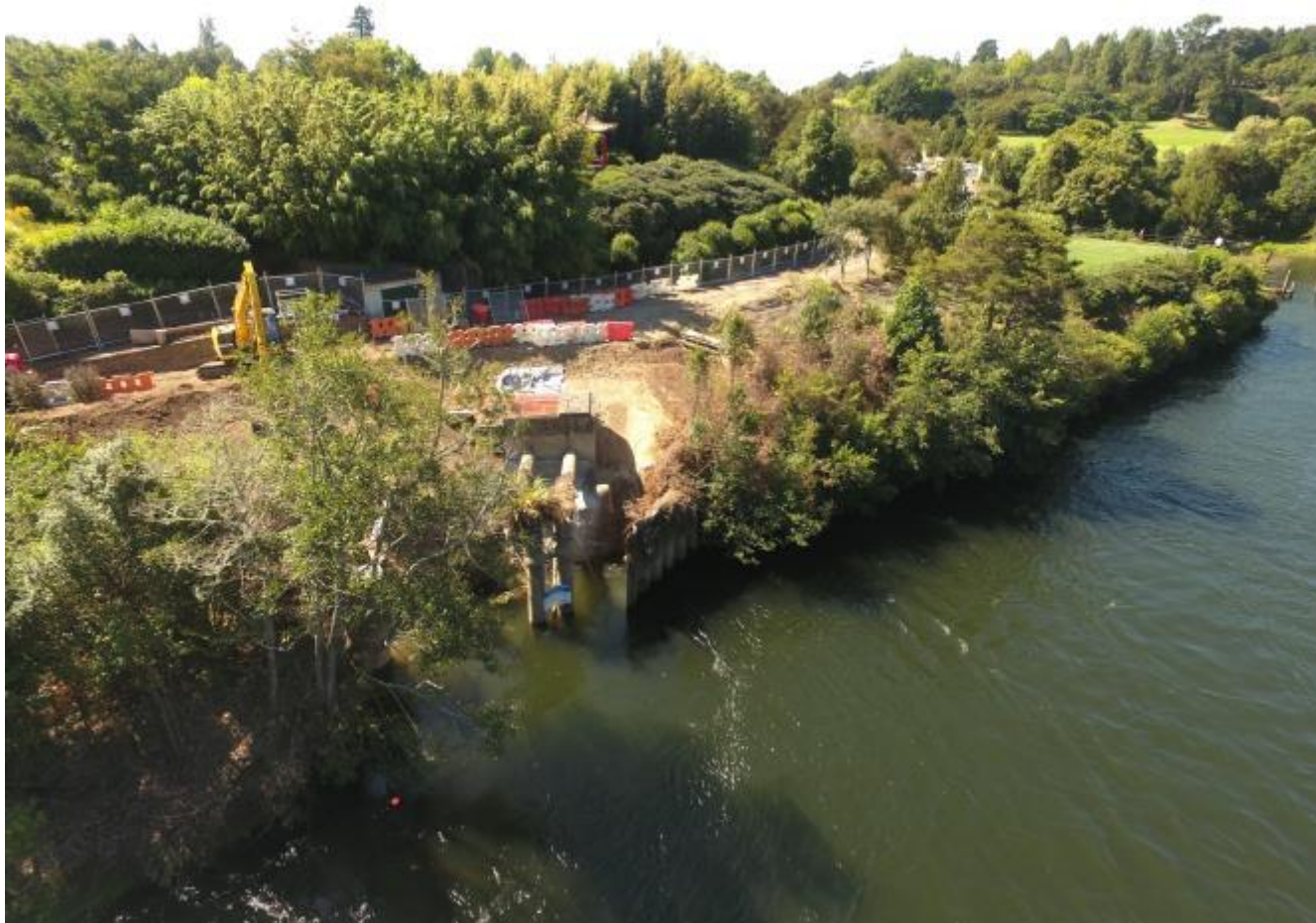
Figure 2. Aerial location of the eastern bulk mains and valve chamber in proximity to Waikato River
