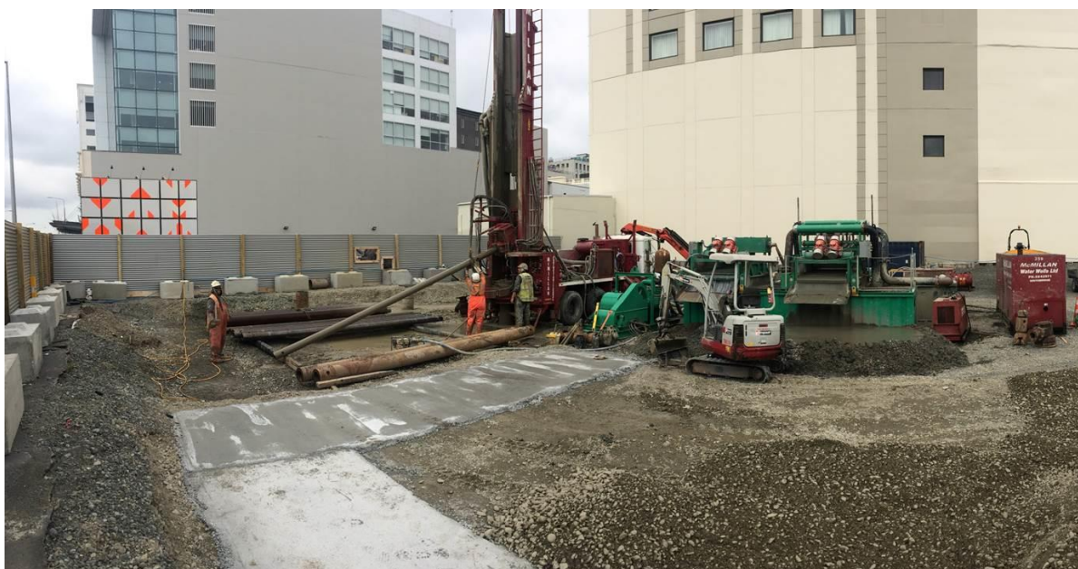
Photograph 3: Dual rotary drilling rig working on an abstraction well in central Christchurch (photo courtesy of McMillan Drilling)
