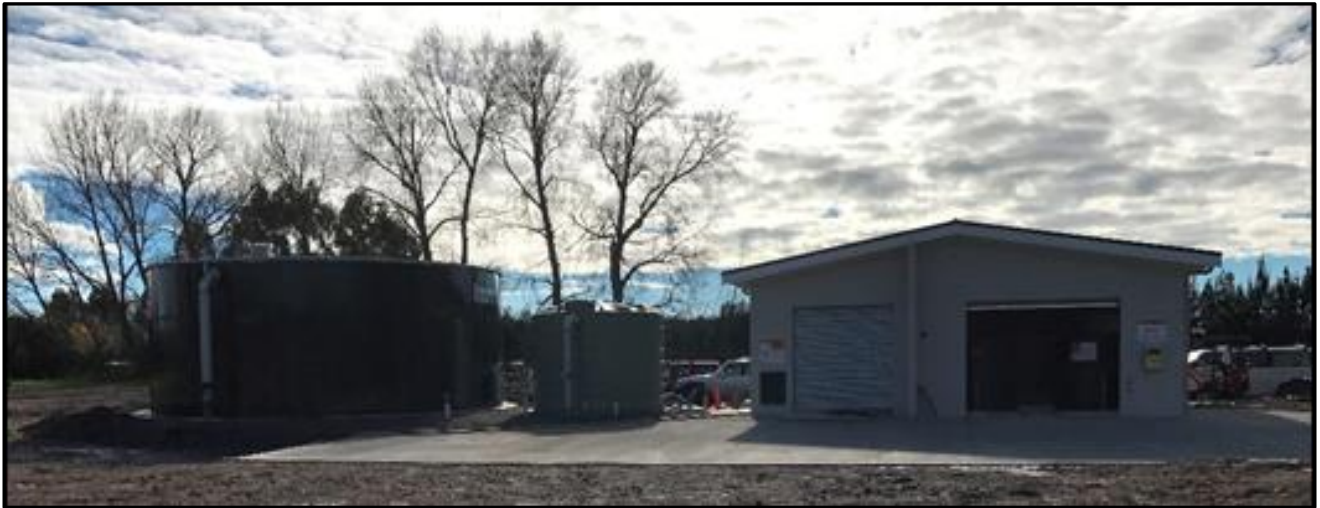
Photograph 2: Otumahi Bore Site Treatment Plant
