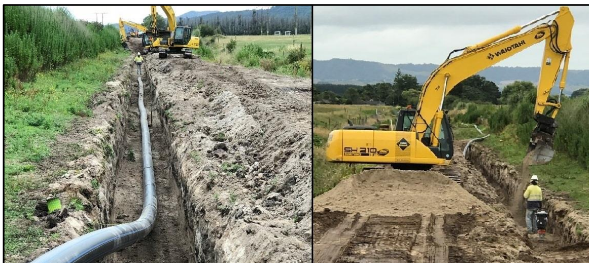
Photograph 1: Otumahi Delivery Pipeline installation
