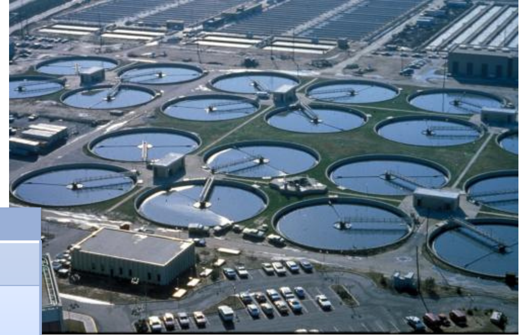
Water Treatment Plant
