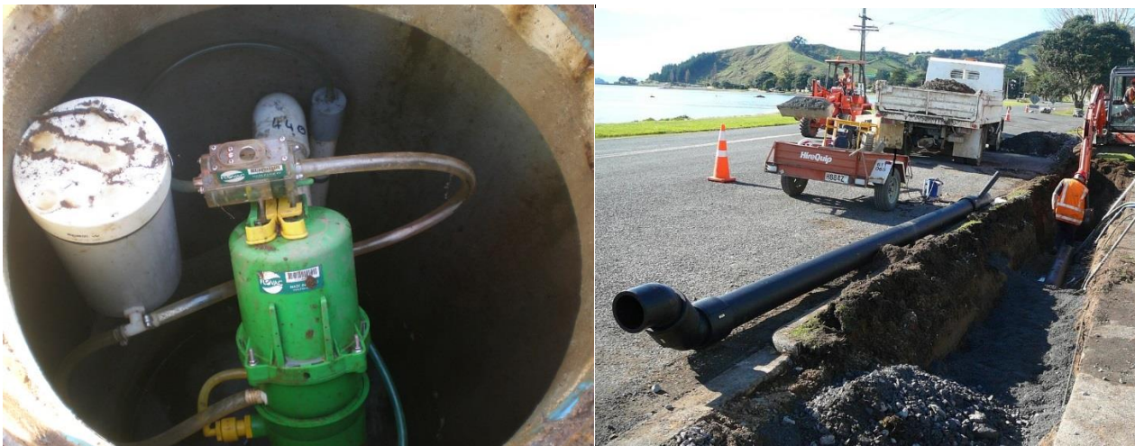
Photograph 1: A Vacuum Pit and Vacuum Sewer Line being installed
