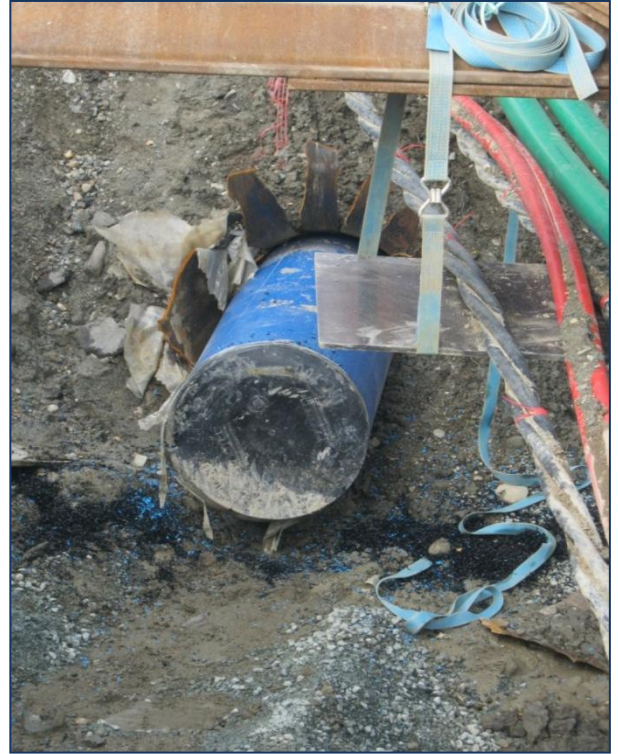
Figure 8. The new main installed after the pulling head had been removed.
