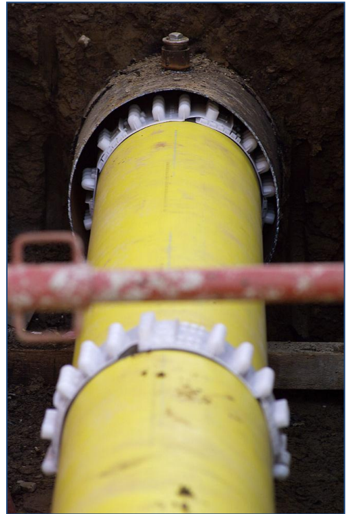
Figure 5. Plastic spacers centralise the PE80 liner in the gas main.
